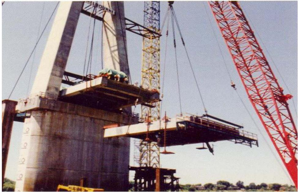
**FIGURE 4: Barge mounted crane hoists 275 ton, pre-cast concrete, deck segment with alignment tongue in view**
