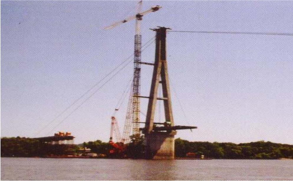
**FIGURE 2: Ohio shoreline view of the guyed, 278.83' tall concrete pylon atop the 87' high, existing, main river pier.**
