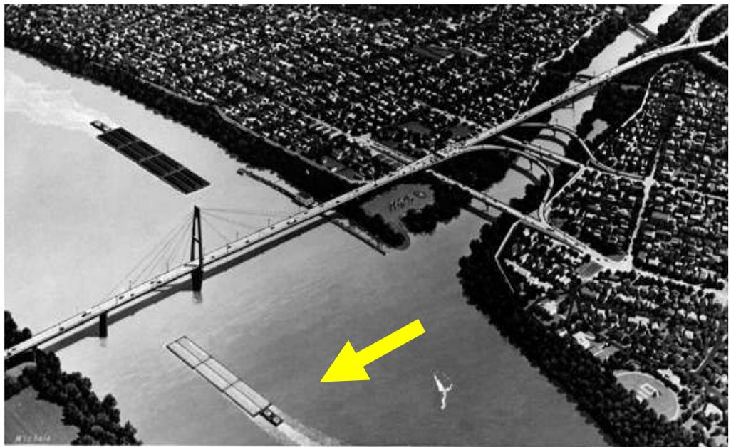
**FIGURE 1: Southeast view of original, mid-stream, pylon location for the East Huntington, steel, cable-stayed bridge**
